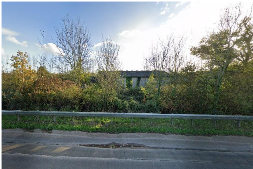
Existing buildings looking south from the A30
